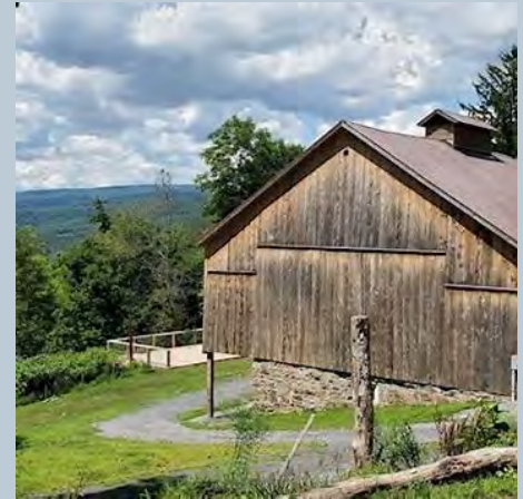
The barn at Evergreen Heritage Center used for events on the upper floor and a living history museum on the lower floor.
